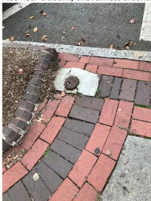
Loose brick at curb between Citibank and Biltmore Tuxedo and large crack/pit filled with water:
