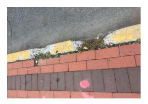
Corner of La Laterna at ramp area. Large space between bricks and curb. Corner of Westside Bagels (tile cracked)
