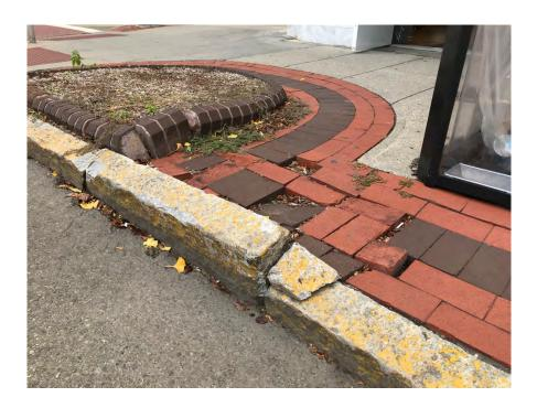
Same corner on curb ramp large deep crack:
